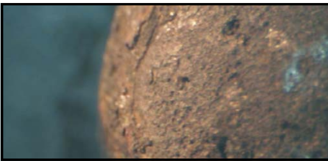
Photo 2. Ball surface after cleaning with corrosion byproducts/magnetite deposits removed.
